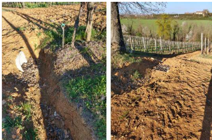
Figure 26: Monitoring of the drain, March 2019
