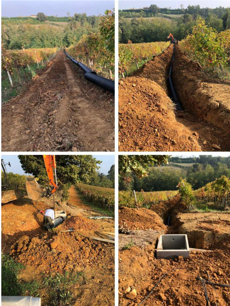
Figure 25: Drainage installation in RES2 demonstrative vineyard in October 2018
